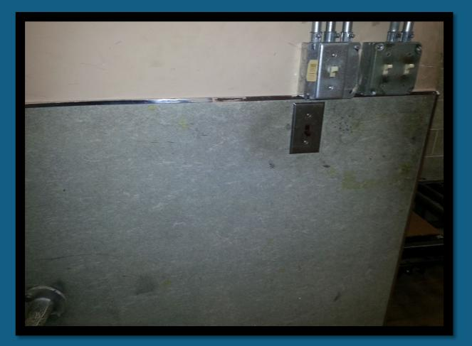
Category II non friable ACMs such as cement siding, Transite board, and shingles, that are subjected to intense weather conditions (thunderstorms, high winds or prolonged exposure to high heat and humidity) may become "weathered" to a point where they become friable.
